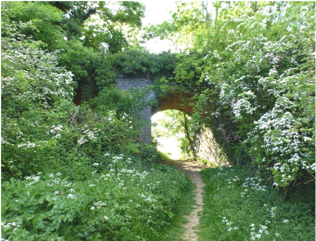
Figure 6 C - Part of the Local Green Space Public footpath under Railway Bridge leading to Welbourn Lower Fields
