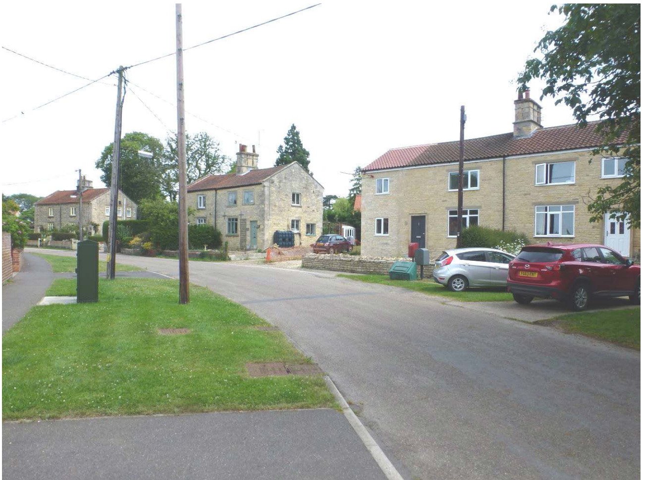
Location 14 – Showing three of the four pairs of semi-detached 19 th century cottages
